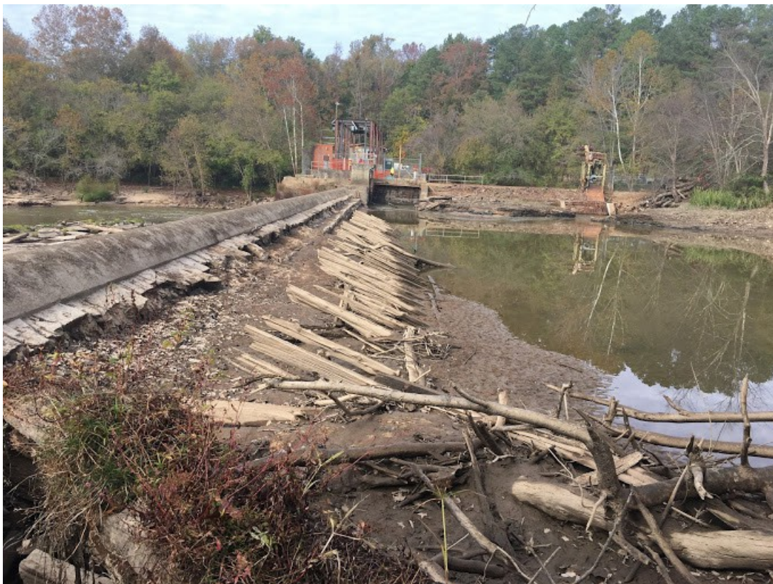
Figure 4: Upstream surface of Milburnie Dam after water level was dropped, November 2017. Note the inclined timbers forming a sloping upstream surface of the dam. These timbers had been submerged for 117 years. (Photo: Courtesy of Restoration Systems.)
